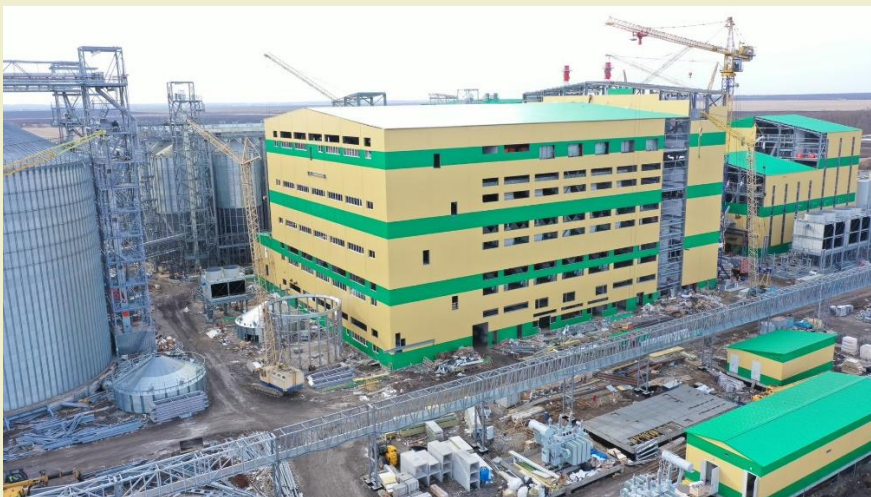
Construction site of Kernel new oil-extraction plant in Western Ukraine, February 2022.
